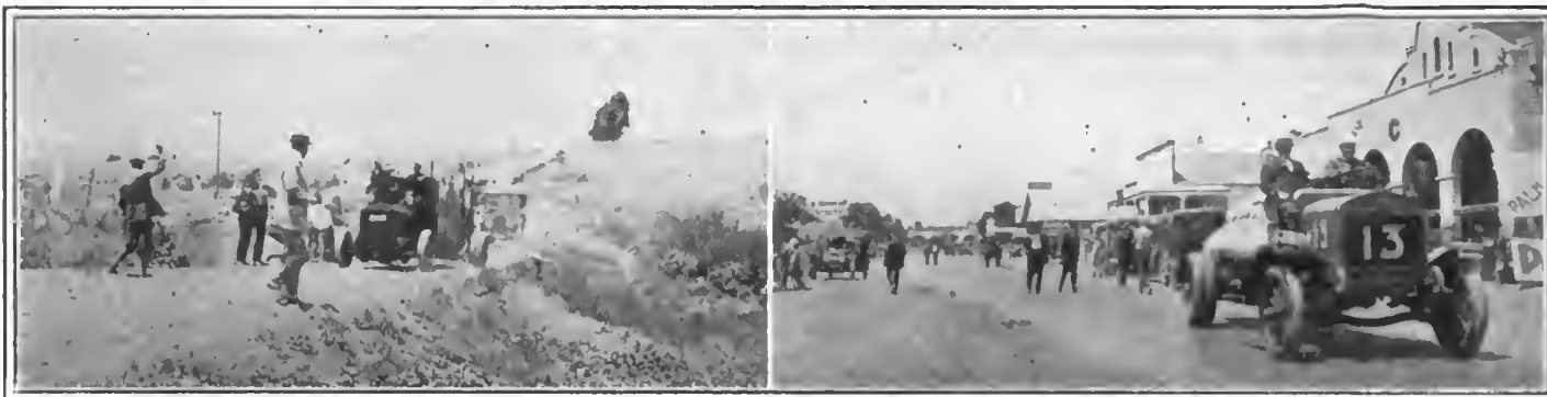
Left—Doane truck crossing frail bridge with 12,000-lb. load in Panama-California Exposition Commercial Vehicle run, Los Angeles to San Diego, July 14 and 15. Right—Trucks checking in at San Juan Capistrano, the first day noon control
